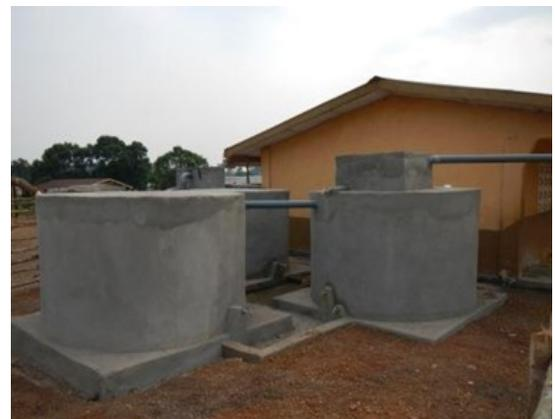
Above is the rainwater harvesting system at Mokonde Primary School. The first-flush diverter is located on top of the far right tank. Photo taken by Jessica Lay.
